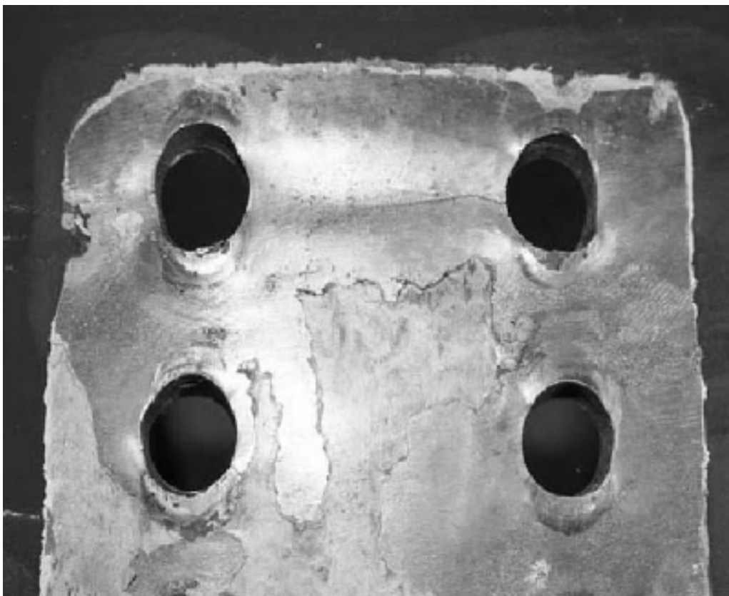
Figure 10.16 Bearing failure of plates
