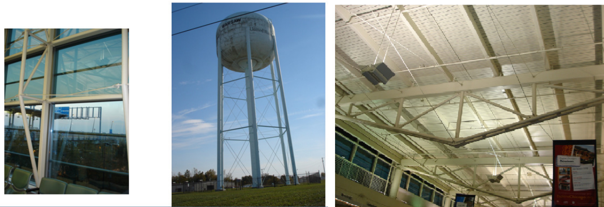
Tie Rods in Structures
